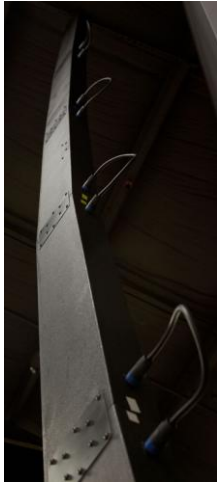
Fig. 18. Back view of array showing side mounting plates and connections between the array wedge boxes with short Speakon cables
